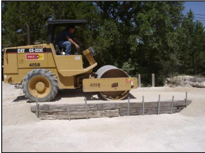
COVER SOIL/AGGREGATE IS UNIFORMLY SPREAD AND COMPACTED USING FIELD-SCALE EQUIPMENT AND PROCEDURES
