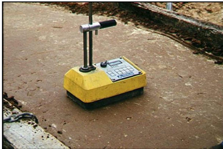
THE DENSITY OF COMPACTED SOIL IS MEASURED
