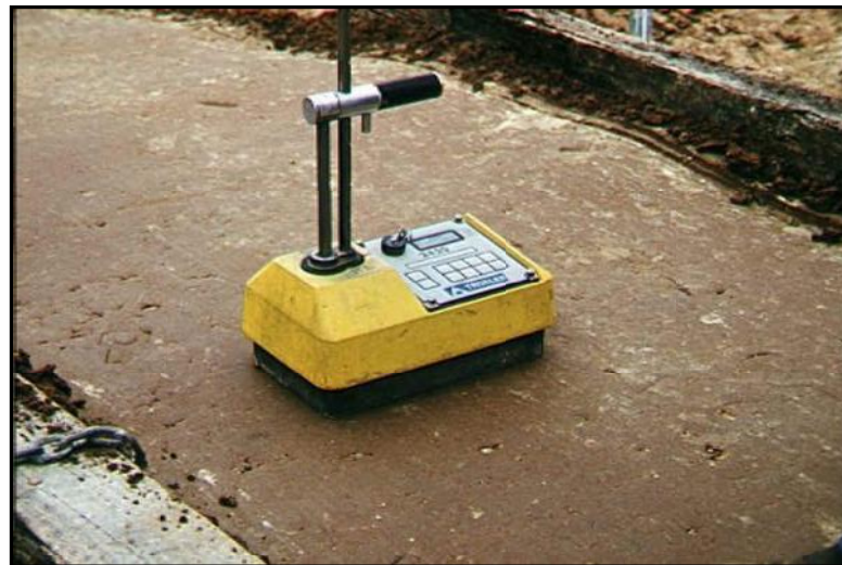
THE DENSITY OF COMPACTED SOIL IS MEASURED
