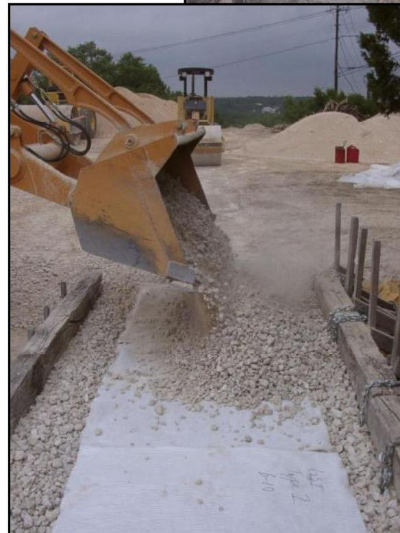
GEOSYNTHETIC POSITIONED OVER COMPACTED BASE AND COVERED
