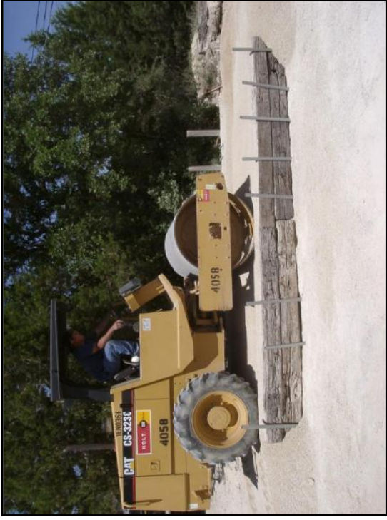
COVER SOIL/AGGREGATE IS UNIFORMLY SPREAD AND COMPACTED USING FIELD-SCALE EQUIPMENT AND PROCEDURES
