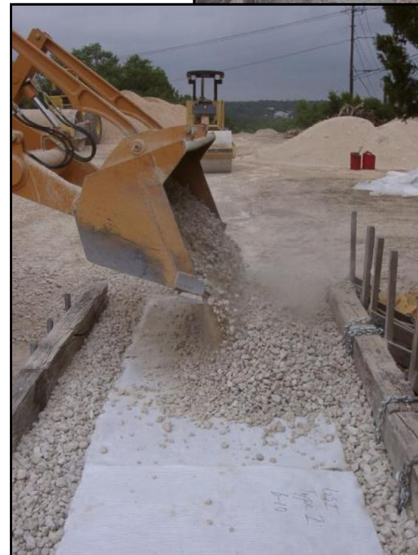
GEOSYNTHETIC POSITIONED OVER COMPACTED BASE AND COVERED
