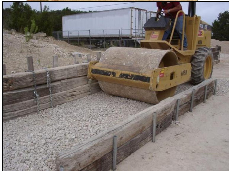
LIFTING PLATES POSITIONED BETWEEN TIES AND COVERED WITH FIRST LIFT OF COMPACTED SOIL/AGGREGATE
