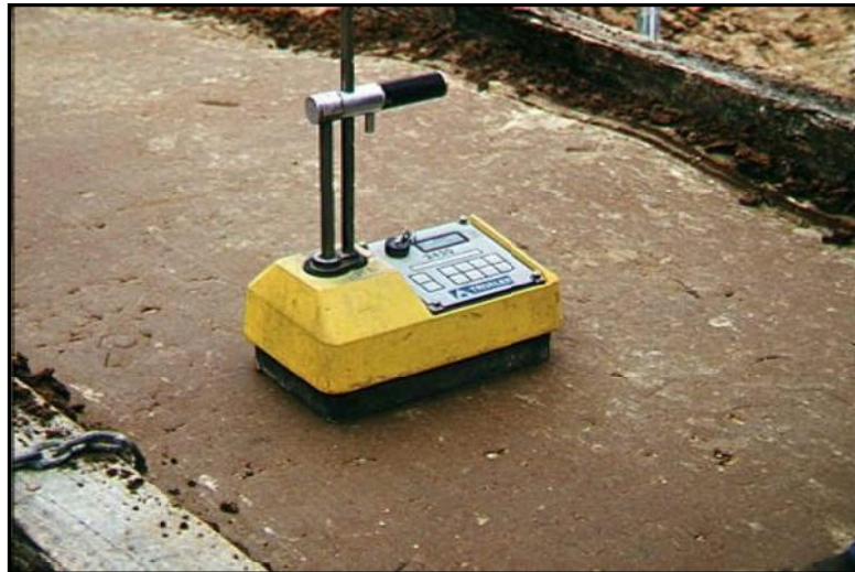
THE DENSITY OF COMPACTED SOIL IS MEASURED
