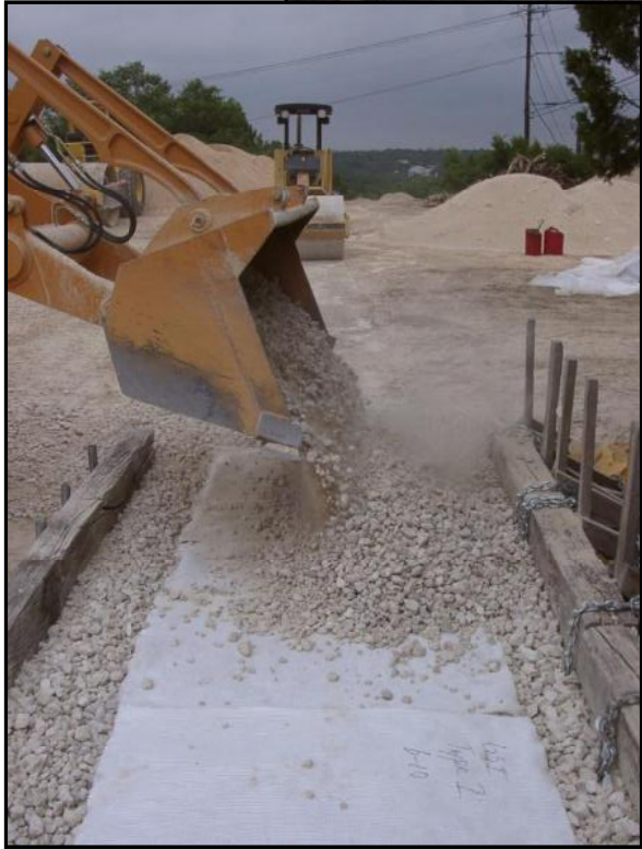
GEOSYNTHETIC POSITIONED OVER COMPACTED BASE AND COVERED
