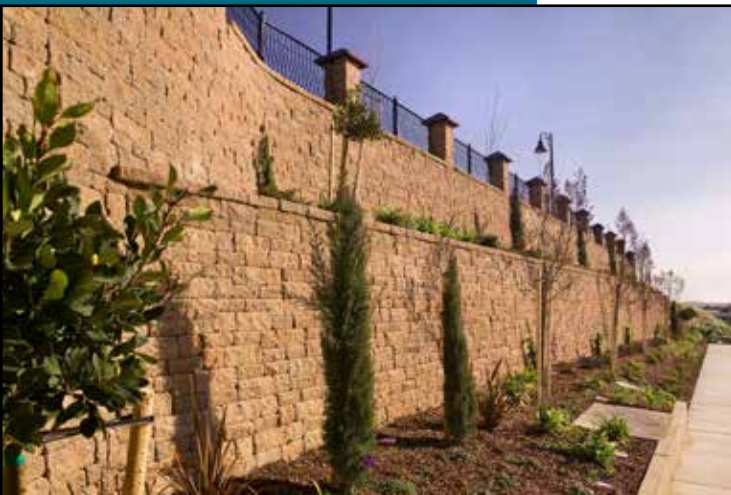
Figure 1. Property Completed and Inspected Wall
