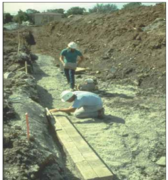
Figure 4. Leveling Pad and First Block Installation
