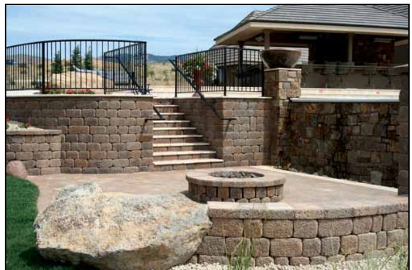
Figure 7. Soft-Slip SRW Facing, Tumbled (Courtesy of Keystone)
