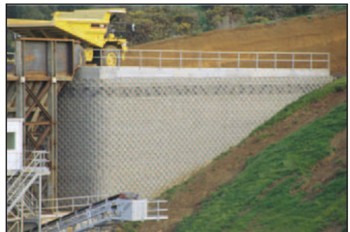
Figure 21. Quarry Support Wall (Courtesy of Keystone Retaining Walls)
