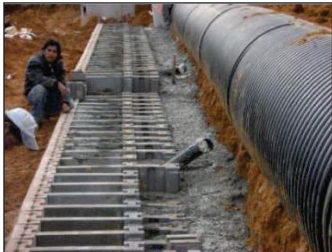
Figure 12. Multi-Depth SRWs (Courtesy of WestBlock Systems, Inc.)
