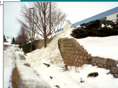
FIGURE 5 SNOW ACCUMULATION ON WALL (REF. 8, FIGURE 4.12)
