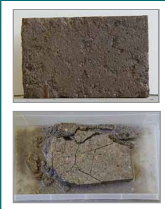
FIGURE 7 SRW SAMPLES SPECIMENS AFTER ASTM C1262 TESTING IN WATER FOR 100 CYCLES (TOP) AND IN SALINE SOLUTION FOR 60 CYCLES (BOTTOM) (REF. 6 FIGURES 221 AND 222)
